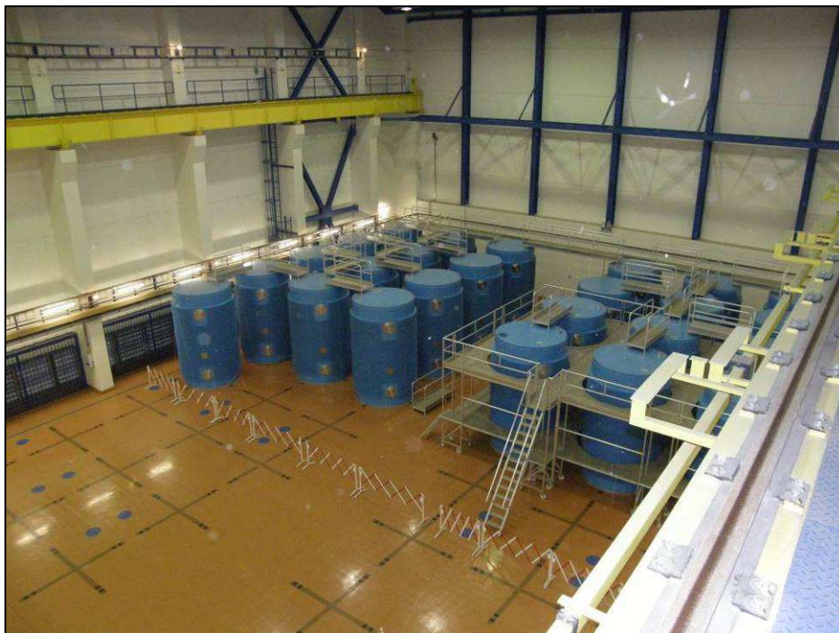
Fig. 4.2 Storage hall in SFSF Dukovany
