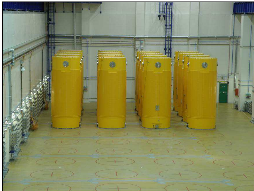
Fig. 4.4 Storage hall in SFSF Temelín
