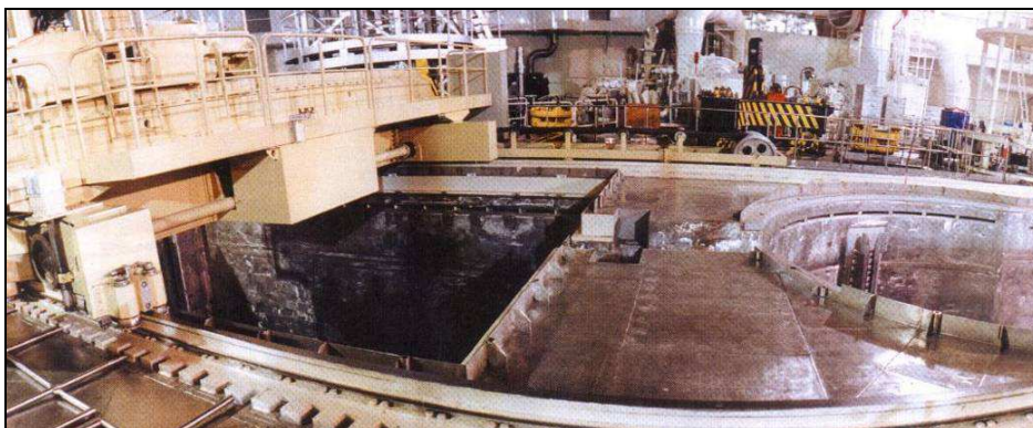
Fig. 4.3 Uncovered SF pool at NPP Temelín
