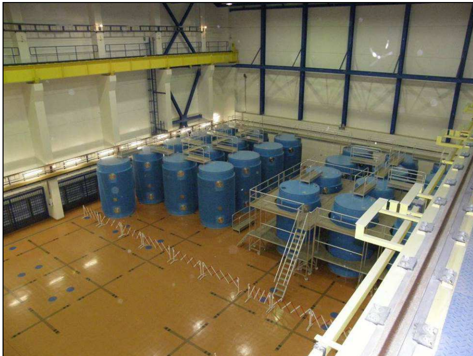
Fig. 4.2 Storage hall in SFSF Dukovany
