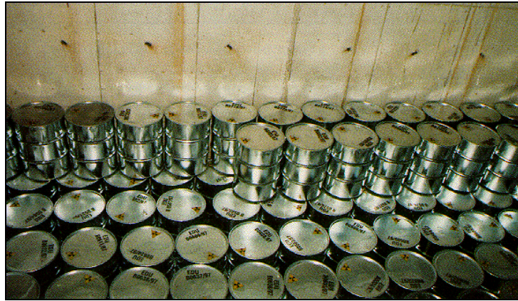
Fig. 8.4 View of a partly filled vault in RAW Disposal Facility Dukovany
