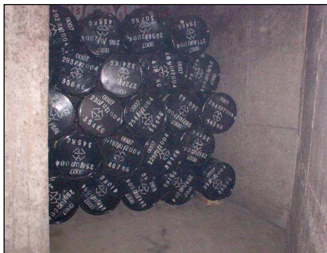
Fig. 8.1 View into a disposal chamber of RAW Disposal Facility Richard
