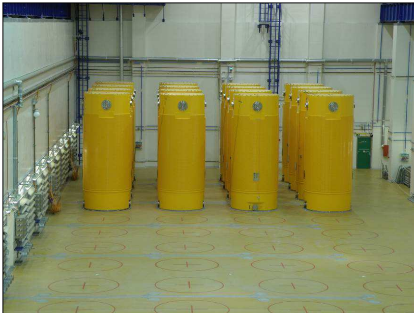
Fig. 4.4 Storage hall in SFSF Temelín
