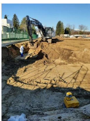
Ispra-Retrieval facility excavation work yard
