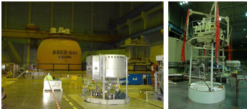
Figure 1: Equipment for decontamination of the primary circuits received at Kozloduy photos SERAW
