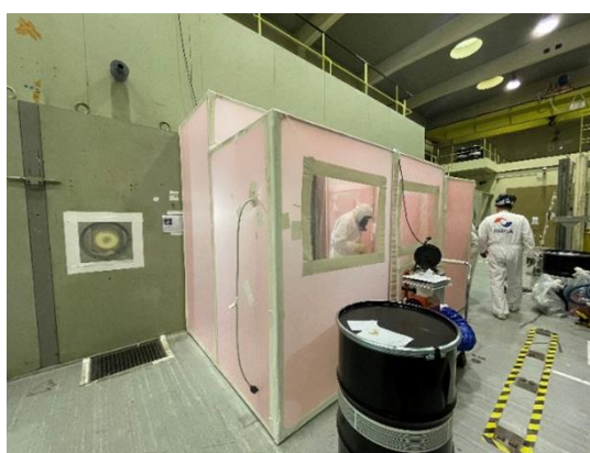
Ispra-Decontamination of hot cells in LCSR
