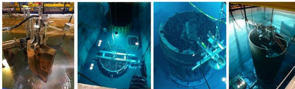
Figure 3: Cutting of Reactor Pressure Vessels at Bohunice
