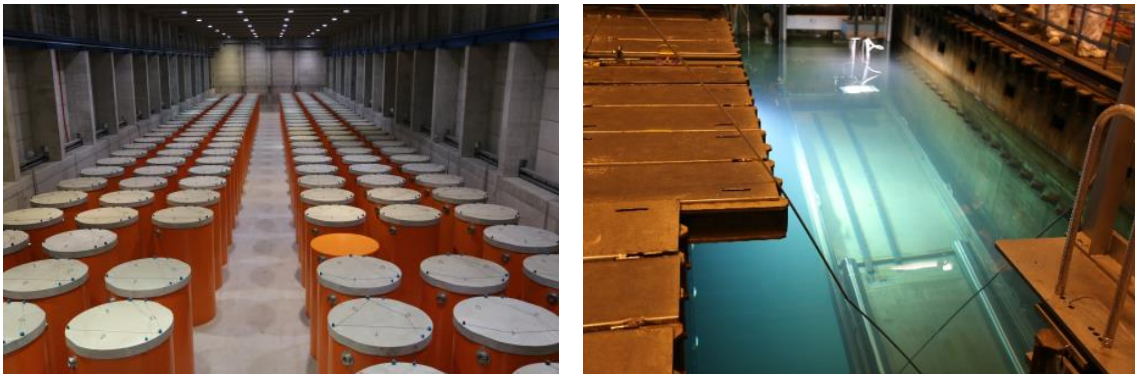
Figure 5: Interim storage facility and underwater cutting of damaged fuel elements at Ignalina photos INPP
